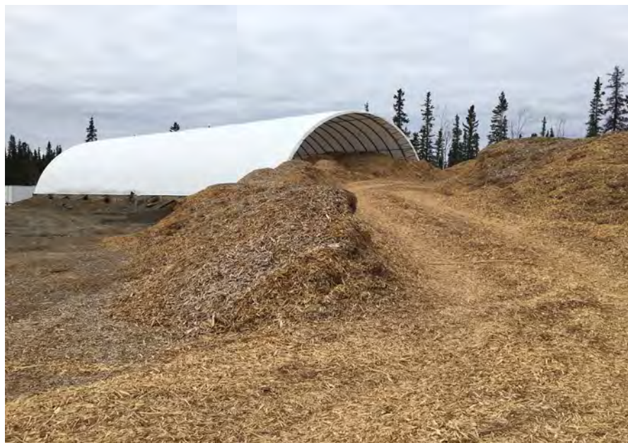
Tok School's shed can hold about 1/7 the chips they need for the year. They are working on getting a timed delivery so their chips do not sit out in the weather.
